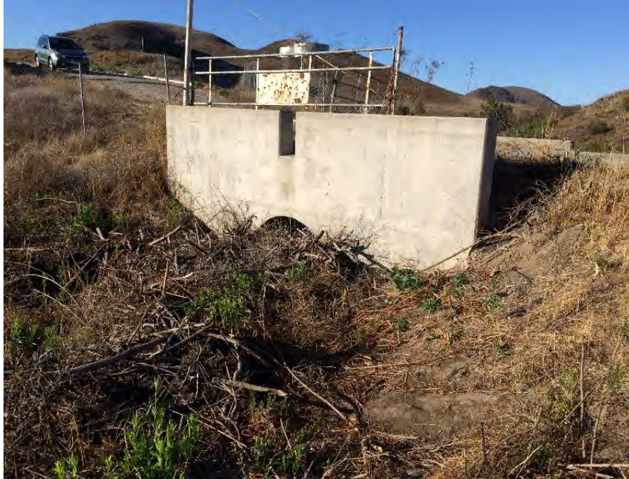
Existing 5' CMP through Inspiration Point Crossing
