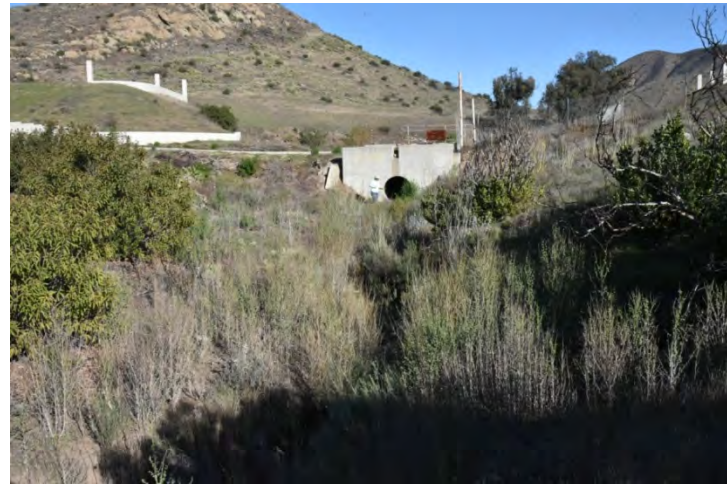
Photograph 4. Typical view of drainage with upland vegetation. View looking east northeast from the western portion of the site.
