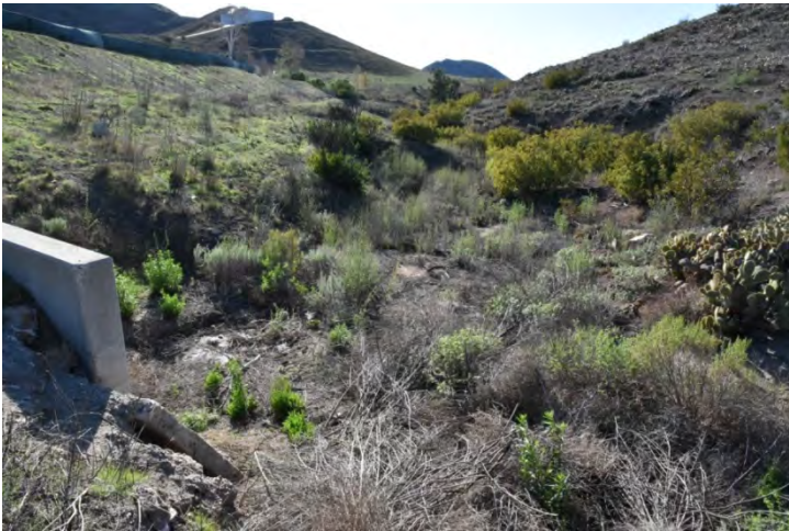
Photograph 3. View facing west southwest. Photo showing current conditions and vegetation west of the culvert.
