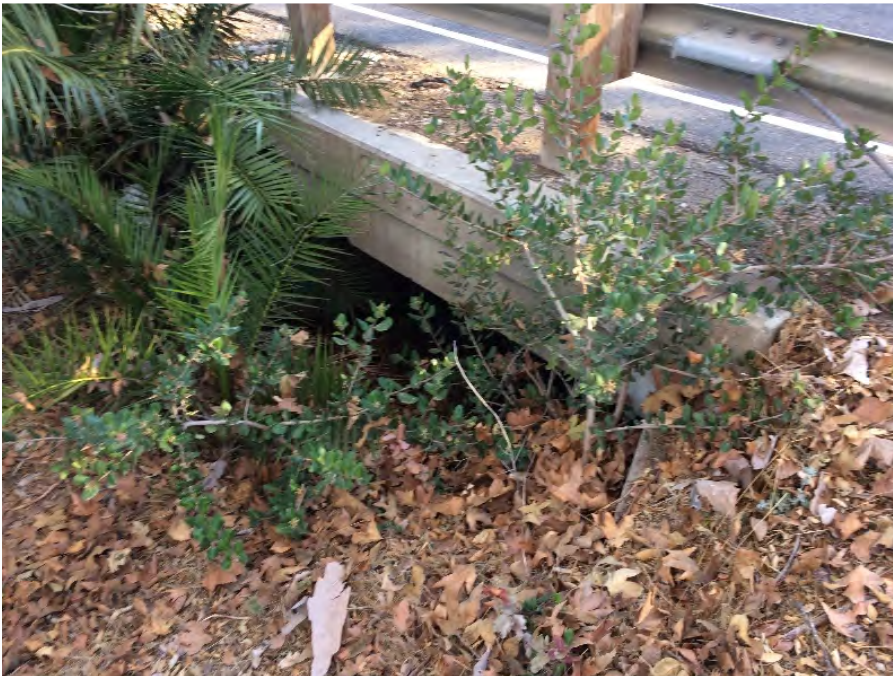
10.3' Long x 2.8' High Rectangular Inlet Structure (10/2016)
