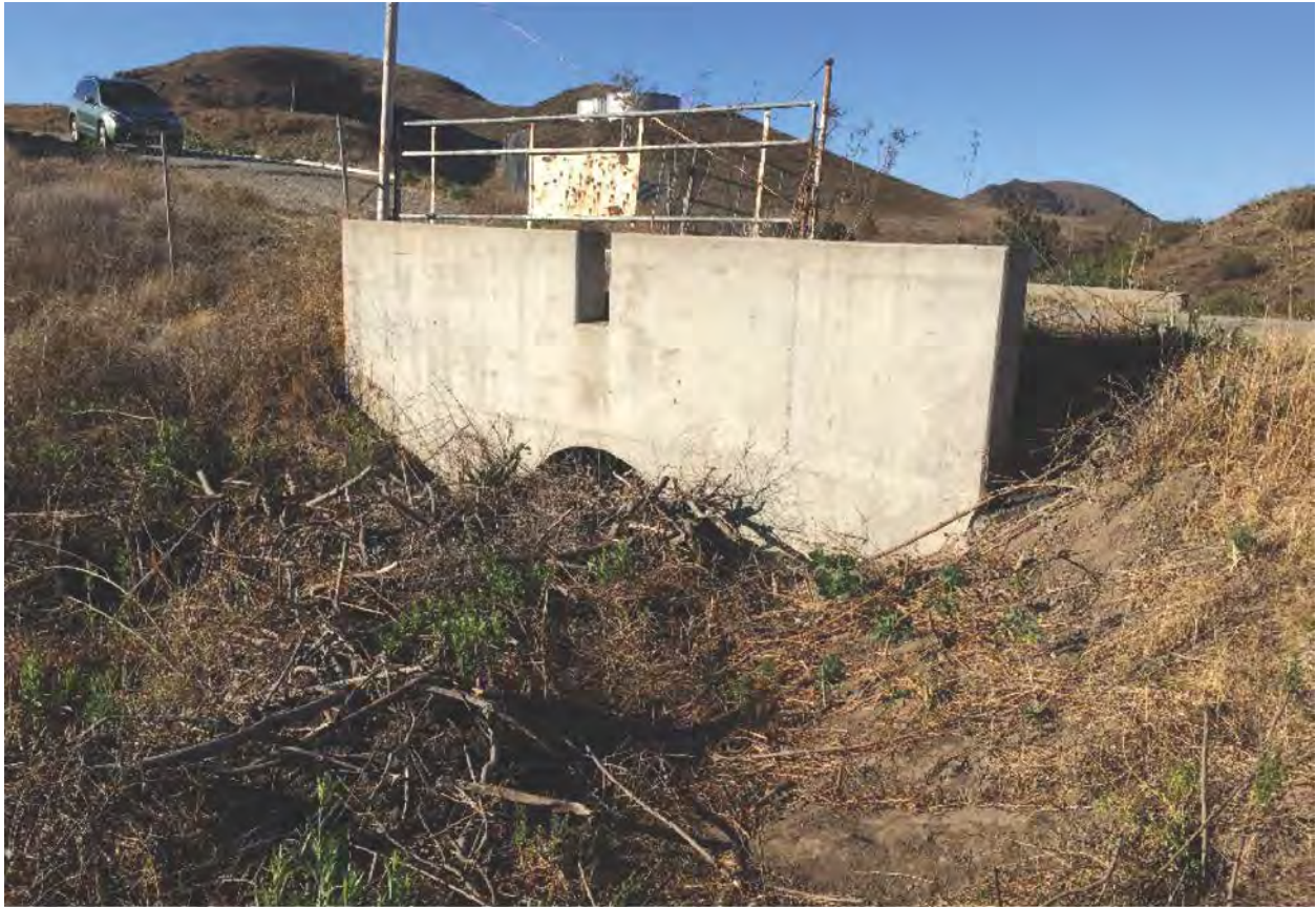
Figure 31 Existing 5-Foot Corrugated Metal Pipe through Inspiration Point Crossing
