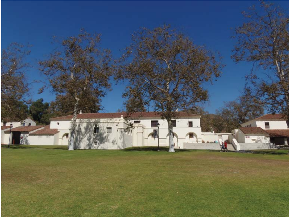
Photo 1: Project site from South Quad.
