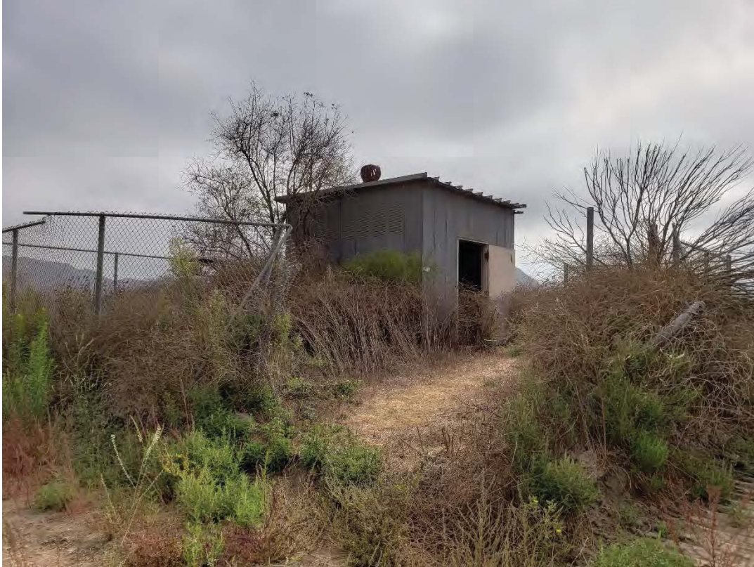
Photograph 5. View of the inactive pump house (to remain) within the project site.
