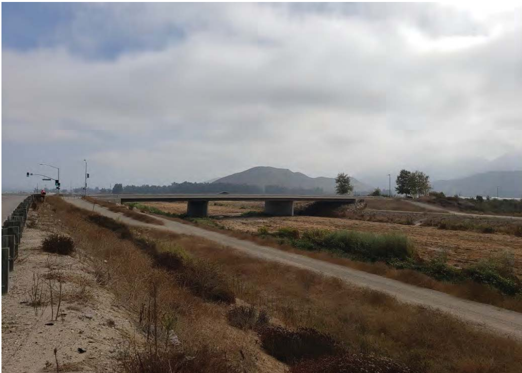
Photograph 6. View northeast from Lewis Road across Calleguas Creek towards intersection of University Drive and Lewis Road, adjacent to the project site.
