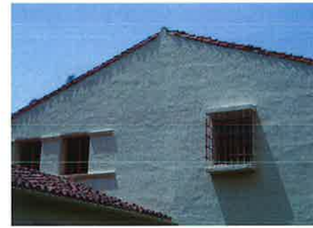
Gable Ends (Note: Tight or No barge)
