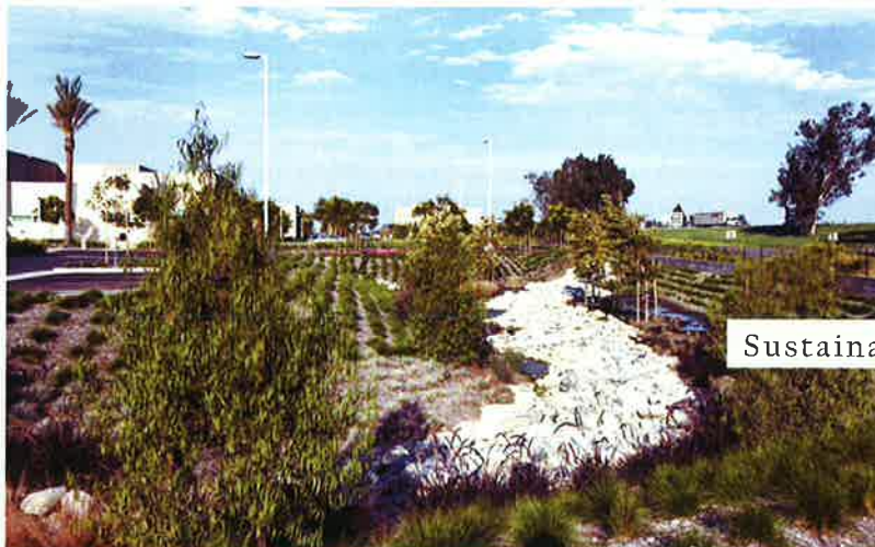
Storm Water Management / Bioswale
