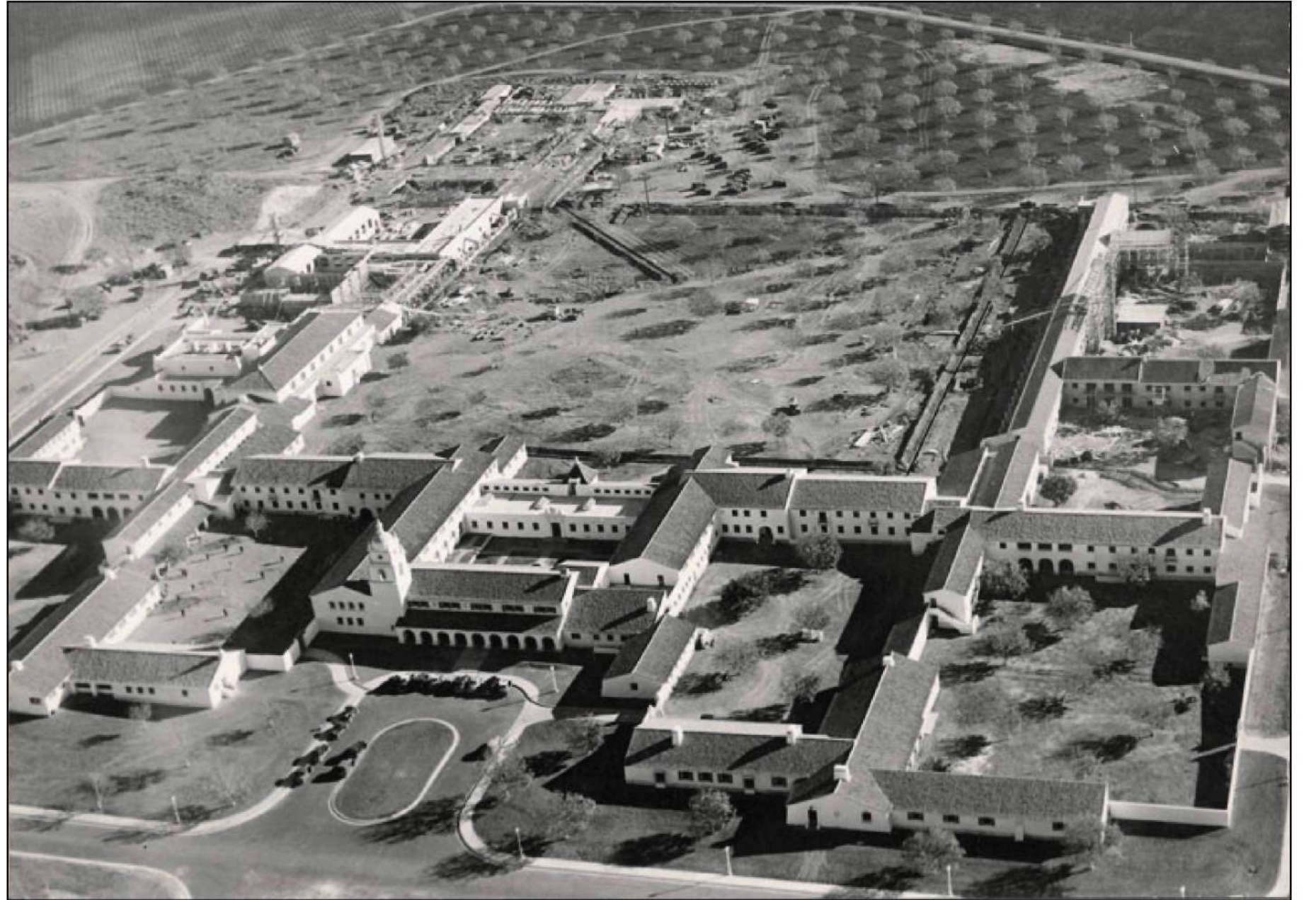
Construction in South Quad, 1937
