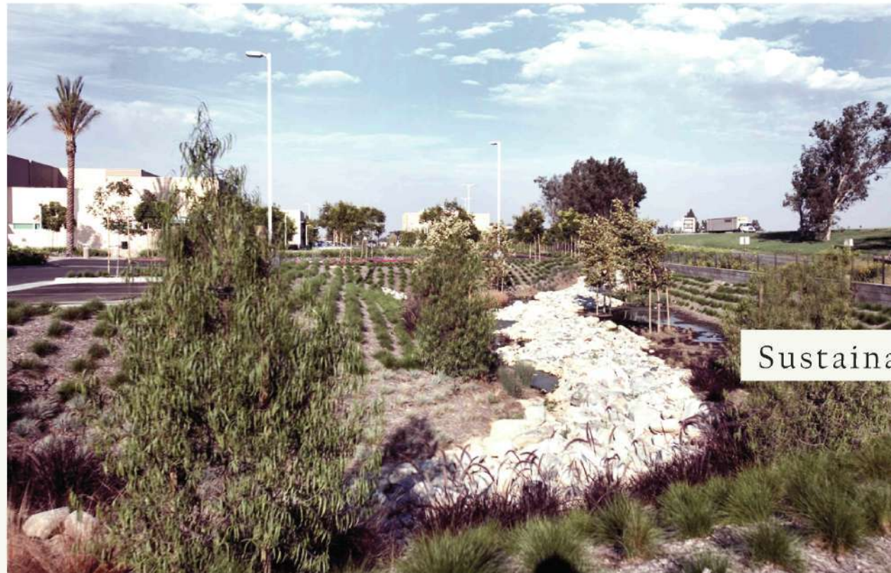
Storm Water Management / Bioswale
