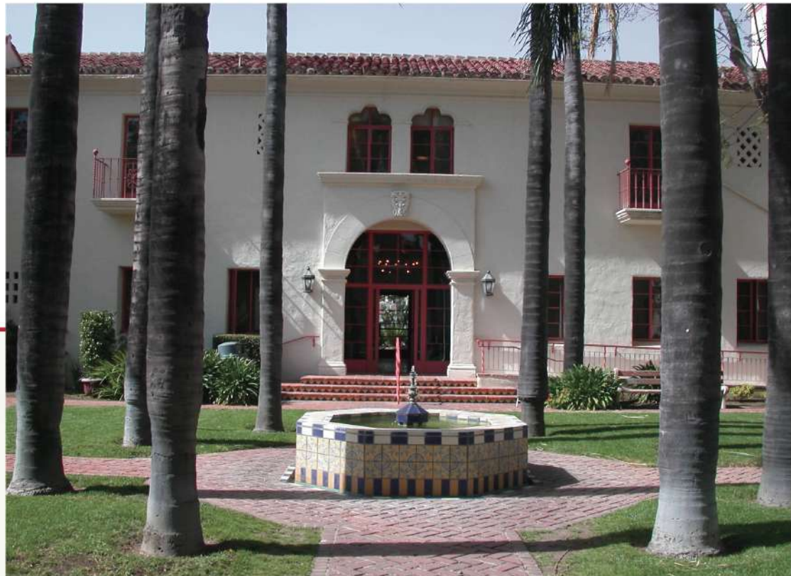
Historic Preservation, retention of mature trees
