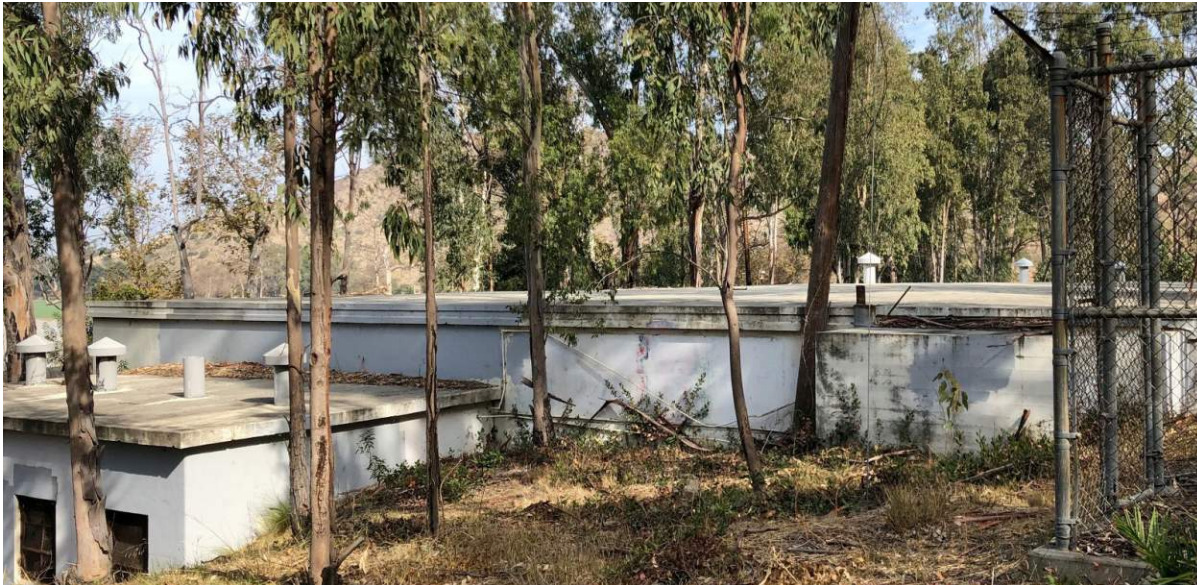
View of Existing Abandoned Buildings on Site M
