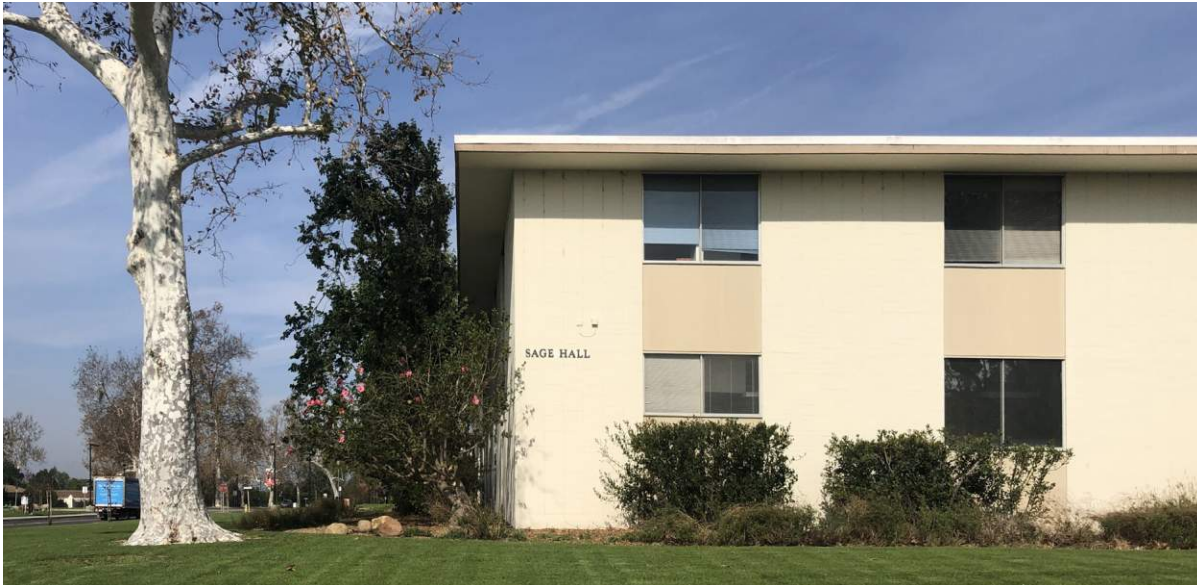
View of Sage Hall which occupies the Northwest Corner of Site G
