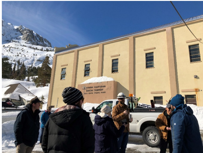
Southern California Edison's Rush Creek hydroelectric plant
