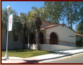
Lindero Hall After Renovation
