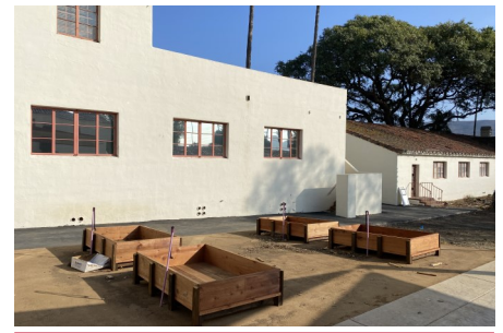
Garden box installation
