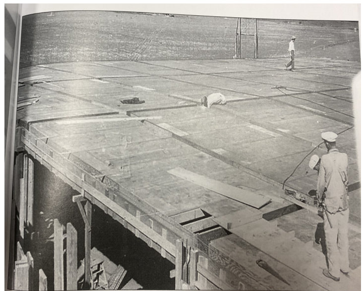
Future hospital bakery under construction (circa 1943)
